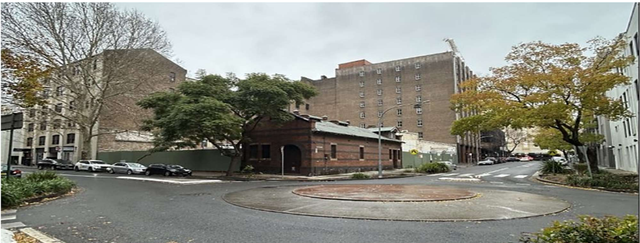
Figure 4 – View southwest towards the corner of Smail and Mountain Streets with the heritage listed electricity Substation in the centre. Adjacent warehouse buildings are located at 55 Mountain Street (left) and 1-3 Smail Street (right).
