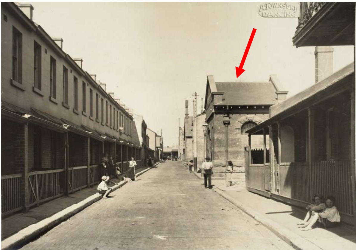
Figure 21 – A photograph dated c.1905 prior to resumption of the Athlone Place area. View from Athlone Place looking south, former 'Substation No.3' is extant on the middle right (red arrow).
